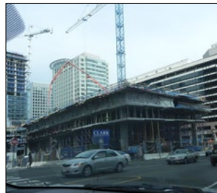
Site Plan #335: Central Place 10,979 sq. ft. retail, 570,549 sq. ft. office, and 9,072 sq. ft. other.
